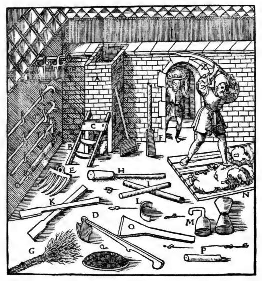
A—FURNACE. B—LADDER. C—BOARD FIXED TO IT. D—HOE. E—FIVE-TOOTHED RAKE. F—WOODEN SPATULA. G—BROOM. H—RAMMER. I—RAMMER, SAME DIAMETER. K—TWO WOODEN SPATULAS. L—CURVED BLADE. M—BRONZE RAMMER. N—ANOTHER BRONZE RAMMER. O—WIDE SPATULA. P—ROD. Q—WICKER BASKET. R—TWO BUCKETS OF LEATHER IN WHICH WATER IS CARRIED FOR PUTTING OUT A CONFLAGRATION, SHOULD THE Officina CATCH FIRE. S—BRASS PUMP WITH WHICH THE WATER IS SQUIRTED OUT. T—TWO HOOKS. V—RAKE. X—WORKMAN BEATING THE CLAY WITH AN IRON IMPLEMENT.
